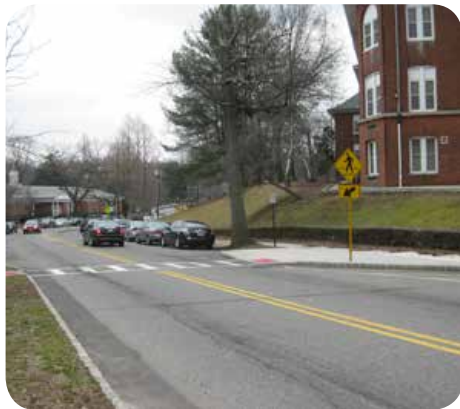
Curb extension in front of the middle school in Maplewood, NJ. Image: The RBA Group
