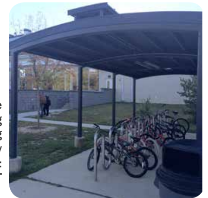
Covered bicycle parking at Egg Harbor's Spragg Elementary School. Image: NJDOT
