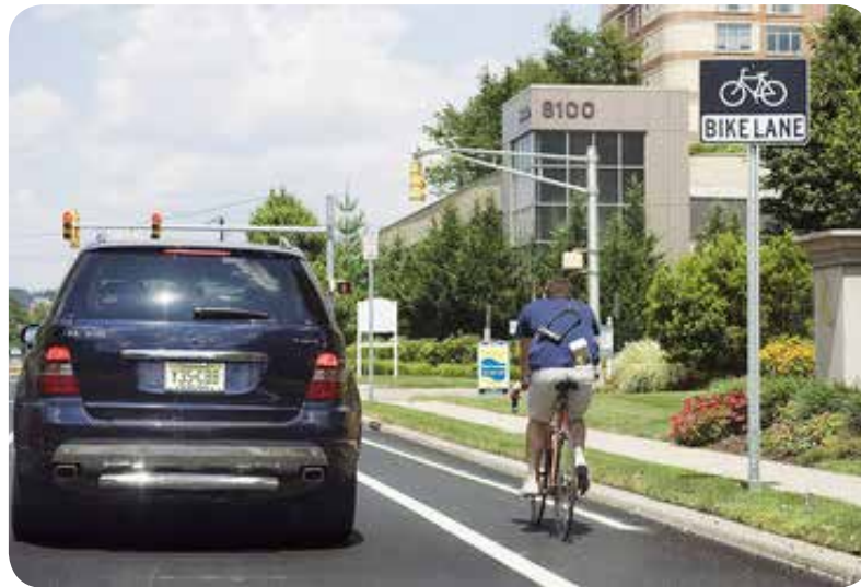
Narrowing the travel lanes on River Road in Hudson County, NJ allowed room for bike lanes. Image: NJ.com
