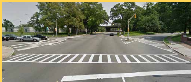
High visibility crosswalks have been installed in the area. In addition, there is no tight turn on red (RTOR) allowed from South Orange Avenue to Oraton Parkway. Image: Google Streetview
