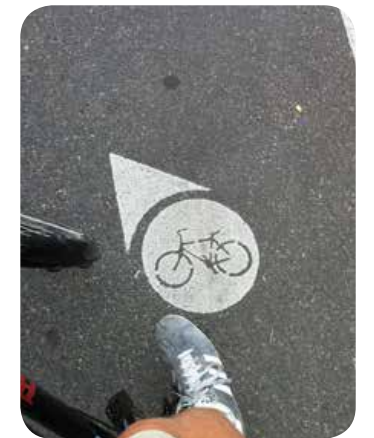
Bike Dots are pavement markings for signed bicycle routes. They are a tool to provide wayfinding. Image: TucsonVelo.com
