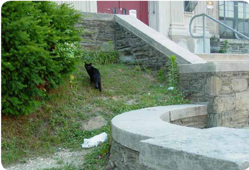
Poor example: This space adjacent to a school building shows signs of wear and offers little in the way of positive activity. Image: The RBA Group
