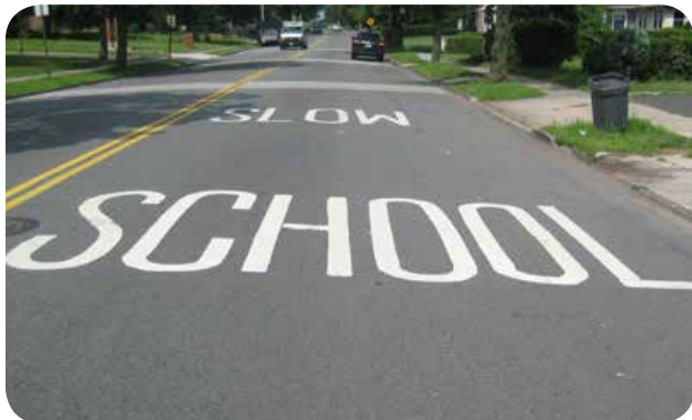
“Slow School” pavement markings on Glenwood Avenue in East Orange, NJ. Image: The RBA Group
