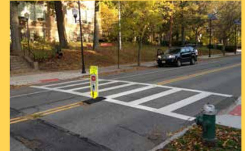
Newly painted high visibility, continental crosswalk and in-pavement “Stop for Pedestrian” crossing sign. Image: Arterial
