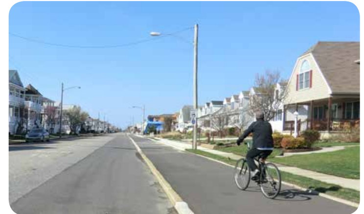
A raised cycle track in Ocean City, NJ. Image: The RBA Group
