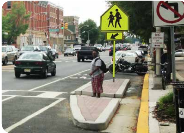
A mid-block storm-water curb extension example, Route 45 in Woodbury, NJ. Image: NJDOT
