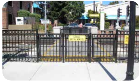
Example of a swing gate. Image: California Public Utilities Commission, Pedestrian-Rail Crossings In California
