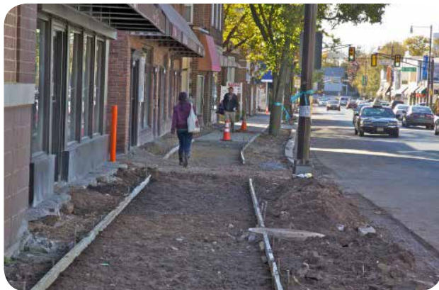
Sidewalk ready to be poured. Image: VTC
