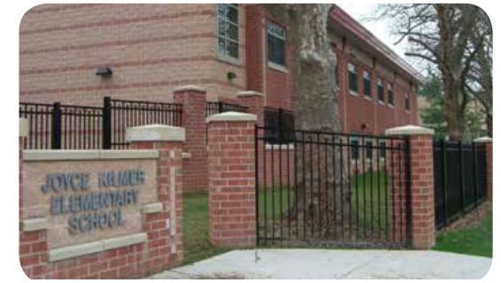
Good example: This painted aluminum fencing mounted on brick piers is both visually permeable and visually appealing. Its integration with the school's sign helps to underscore the importance of the school as an institution and a community. Image: The RBA Group
