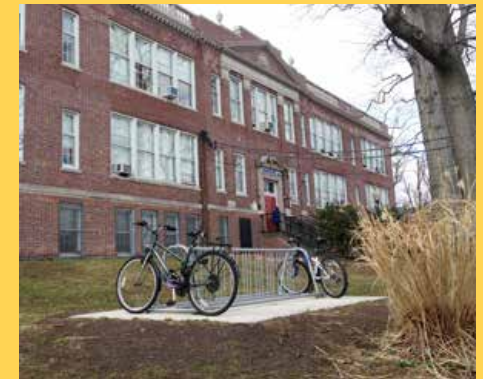
Newly installed concrete pad and bike rack at the front entrance of the school. Image: Arterial
