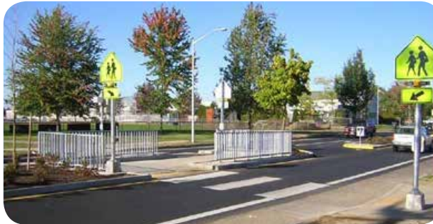
A median with a staggered crosswalk forces pedestrians to turn and face oncoming traffic before crossing the second half of the crosswalk. In order to curtail shortcutting and force pedestrians to follow the intended path, some medians may also have attractive fencing to corral pedestrians in the correct direction. Image: Oregon Department of Transportation
