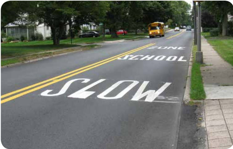
SLOW SCHOOL ZONE pavement marking in Ridgewood, NJ. Image: The RBA Group
