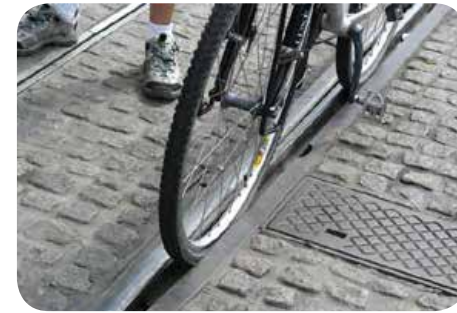
Bicycle tires can get stuck on the grooves between tracks. The safest way to cross rail tracks is as close as possible to a 90 degree angle. Image: BicycleGermany.com
