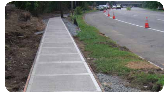
New sidewalk. Image: VTC
