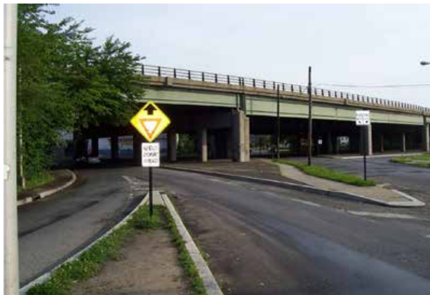
The crosswalks are unmarked and curb ramps absent at this ramp, located one block from an elementary school in Camden. Image: Cambridge Systematics
