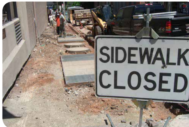
Sidewalk closed for repairs. Image: VTC
