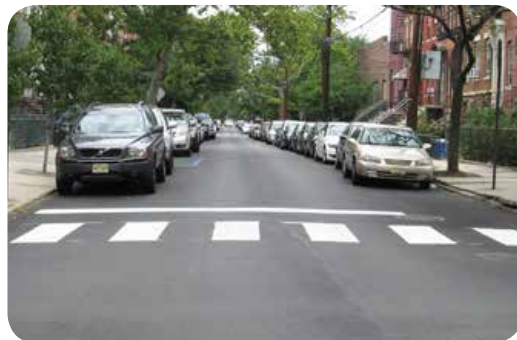
Bar style crosswalk in Hoboken, NJ. Image: The RBA Group
