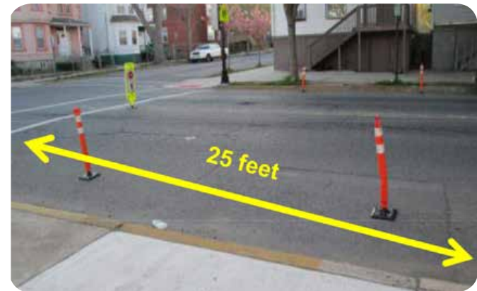
The City of New Brunswick has begun installing plastic pylons in the no-parking area, a practice called “daylighting.” The cost of purchasing and installing the standard-use pylons is minimal and can be done in-house with little delay. Image: VTC
